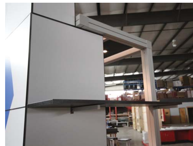
STEP 3: ATTACH THE QUADS AS SHOWN WITH THE NOTCH FOR THE SHELF BRACKET. PLACE SHELVES ON BRACKETS AS SHOWN.
