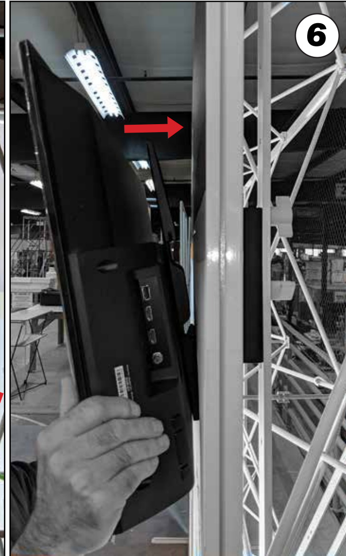
STEPS 6 THRU 8 - HANG TV ON MOUNT THROUGH OPEN AREA IN FABRICS SHOWN
