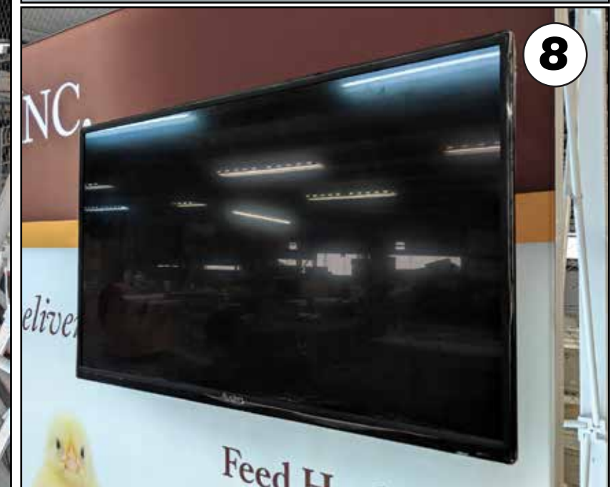
STEPS 6 THRU 8 - HANG TV ON MOUNT THROUGH OPEN AREA IN FABRICS SHOWN
